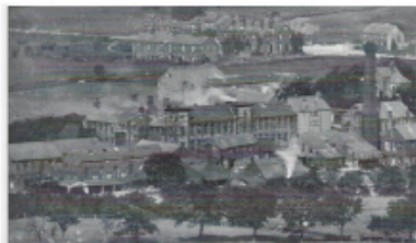
Ecklands Bridge Works
