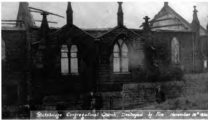
Congregational Church after the fire of November 16th 1921
