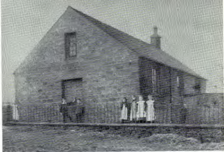
(2) Infant School built in 1853. (From an old photograph).
